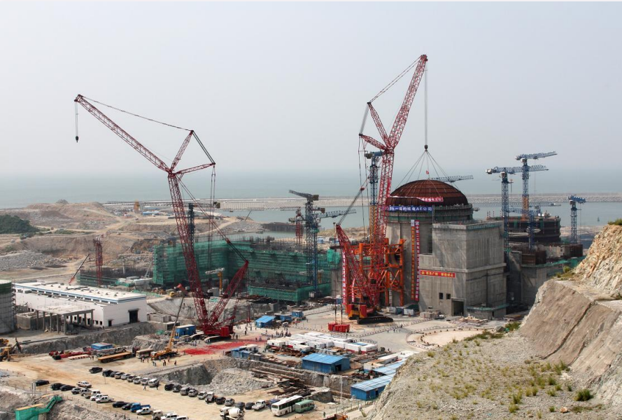
← Yangjiang Unit 1 dome handling
